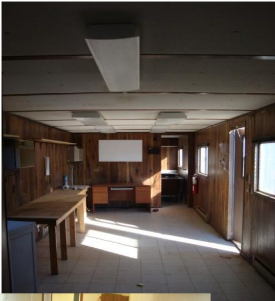
Before restoration of interior Chapel
